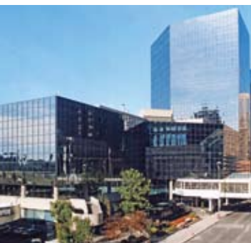
Gulf Canada Square Calgary, Alberta Owner: Great West Life Assurance Company/London Life Insurance Company Manager: GWL Realty Advisors Inc. Architect: K.R. Cooper and Canada Square Corporation
